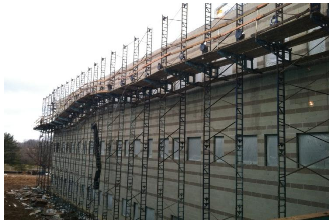
Figure 2: Classroom Wing GF CMU Facade
