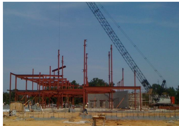
Figure 8: Steel Erection in Section F
