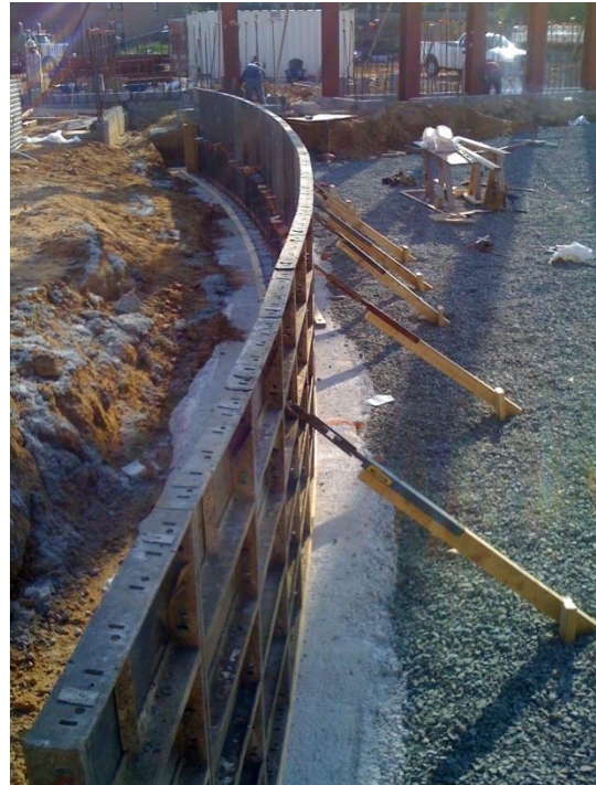
Figure 9: Auditorium Form Work @ Stage Wall
